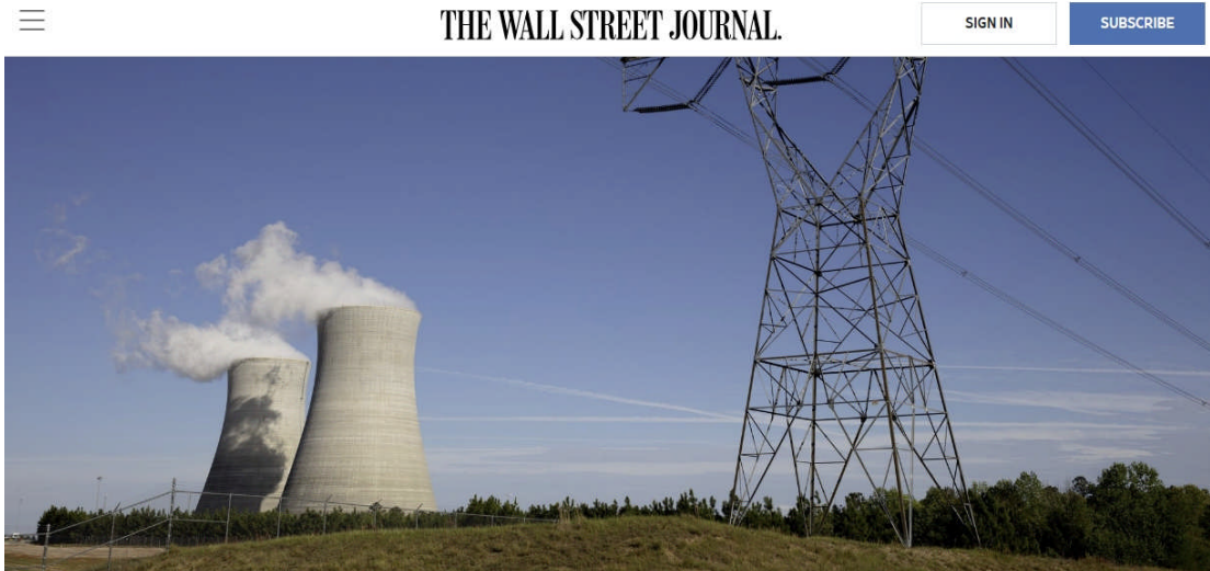
Cooling towers at Plant Vogtle, a nuclear power station in Waynesboro, Ga. KENDRICK BRINSON FOR THE WALL STREET JOURNAL
